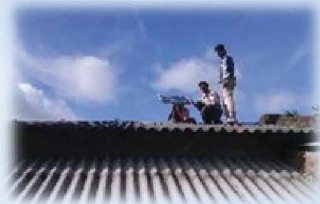
Solar Power Plants
